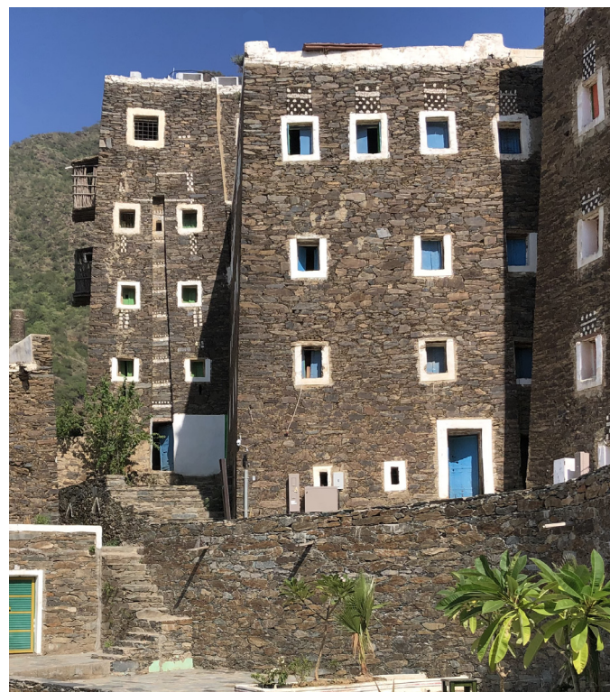
FIG. 20 Vernacular architecture in the Aseer Escarpment
