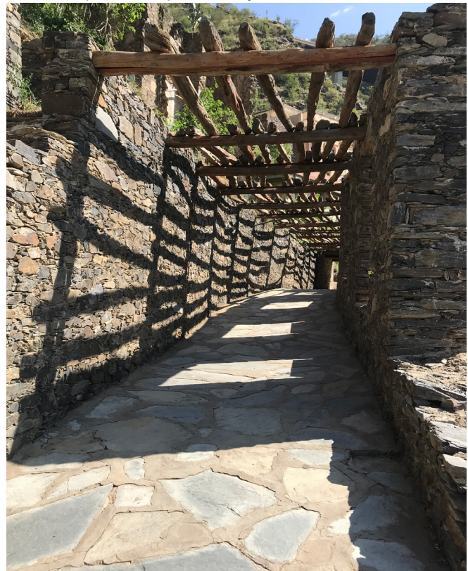
FIG. 67 Shading structure utilizing available natural and local materials. Rijal Almaa, KSA
