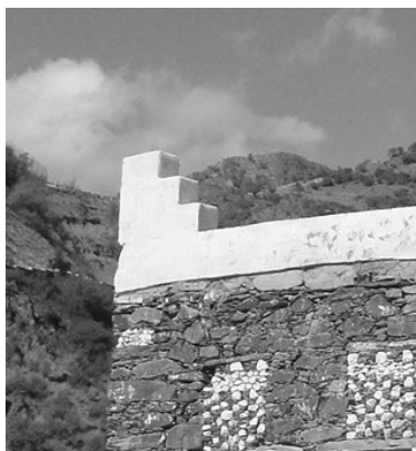
Highlighted stepped parapet
