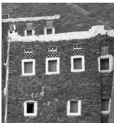
Highlighted parapet banding
