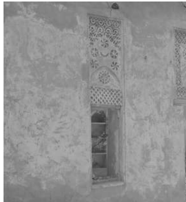
Recess on top of window with articulation
