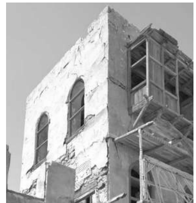
Arch shaped openings
