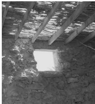
Small ventilation openings
