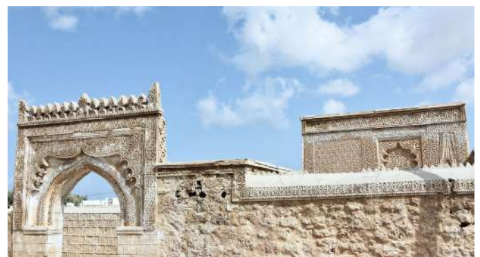
FIG. 19 Example of Farasan vernacular architecture, houses of pearl merchants in Farasan village
