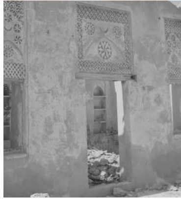
Simple entrance with articulated niche on top
