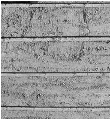
Rammed earth pattern
