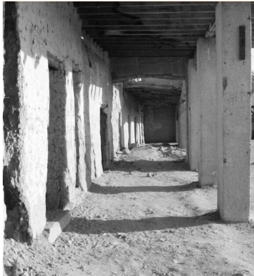
Recessed shading structure on ground floor
