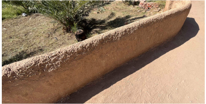
FIG. 65 Retaining boundary walls utilizing natural and local materials such as clay and earth. Al Ula, KSA
